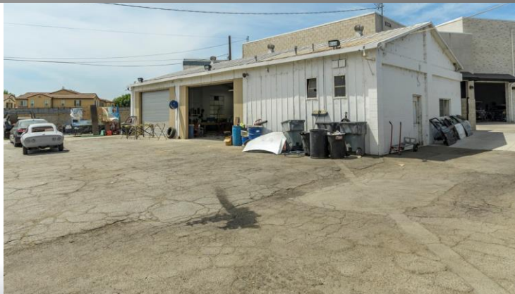
Metal Building for Heavy Repairs
