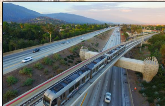
GOLD LINE OVERPASS
